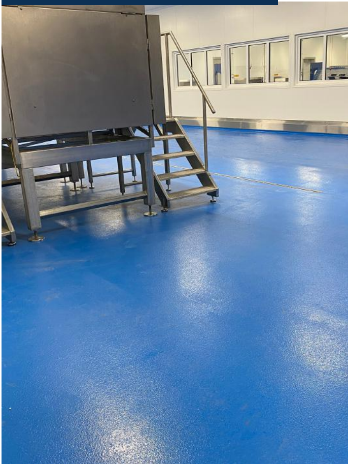
3010 m 2 Stonclad UR was installed
